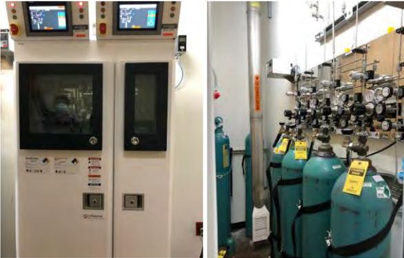
The facility leverages a toxic gas monitoring system that was regularly generating false alarms due to undesirable network traffic.
